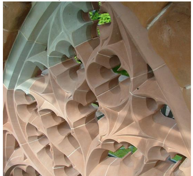
New Tracery after completion (Rear view)
